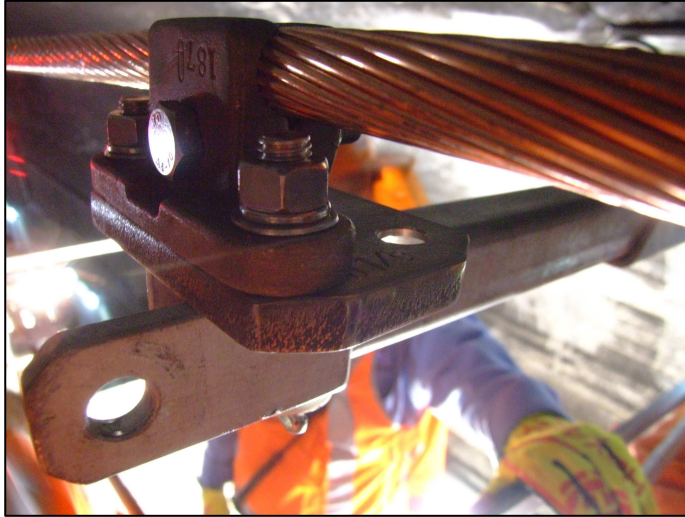
Figure 9 - Catenary Clamp Installed on Swivel Plate
