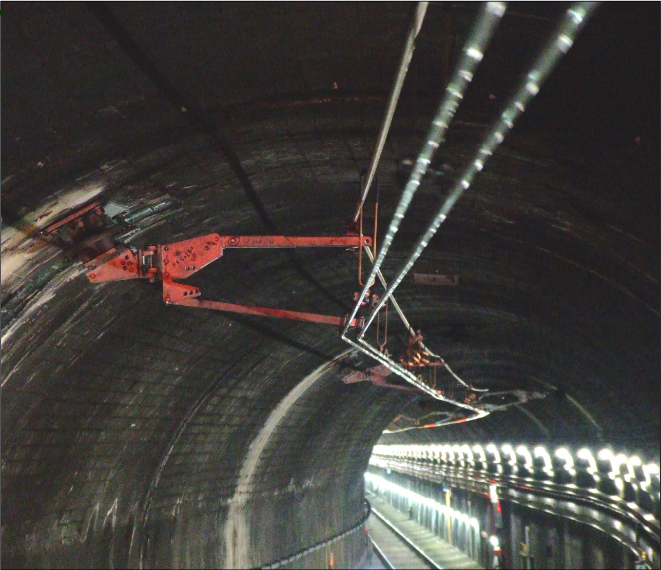
Figure 33 - Mk-3 Tunnel Cantilevers Supporting OHW Around Reverse Trackwork
