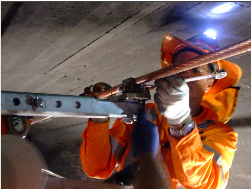
Figure 32 - Tunnel Cantilever Inspections
