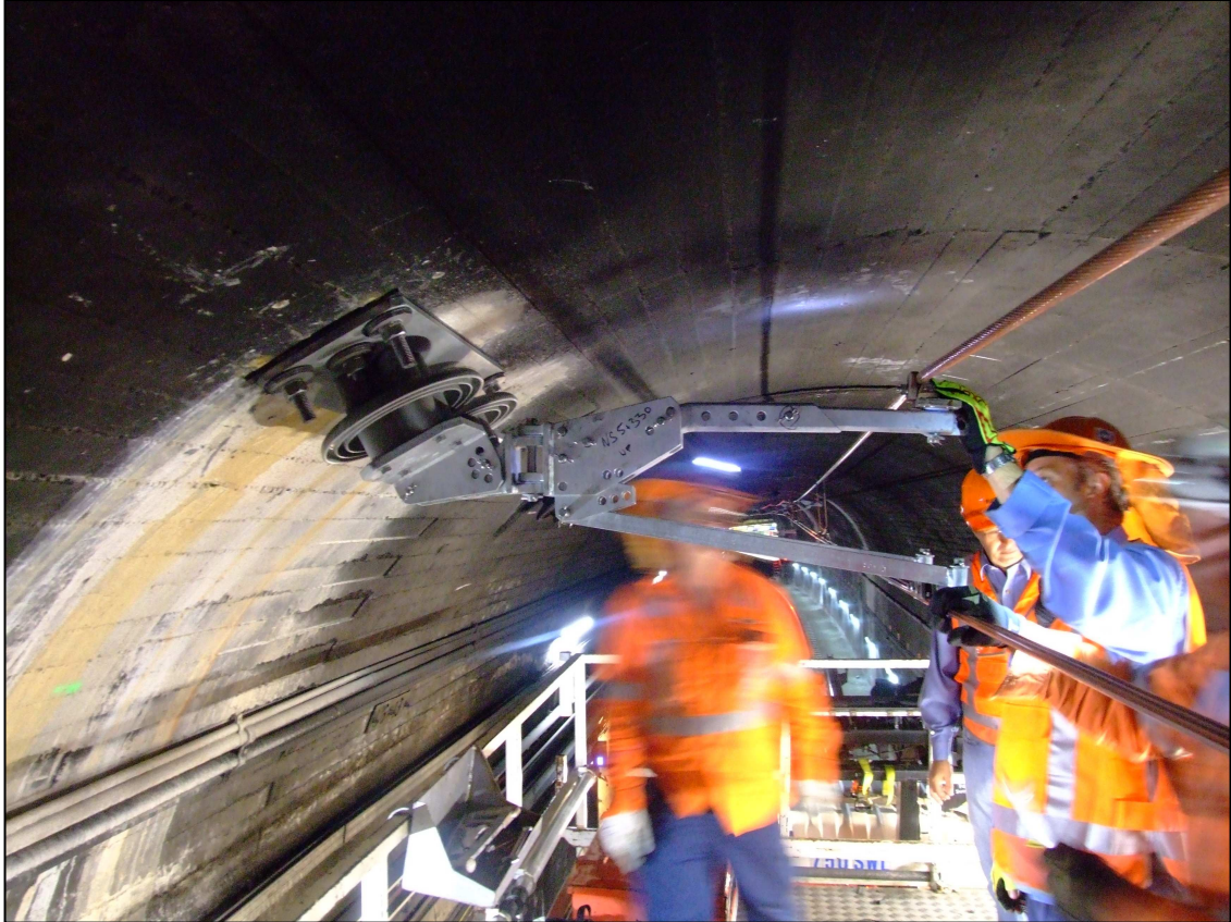
Figure 10 - Installed Tunnel Cantilever Being Adjusted
