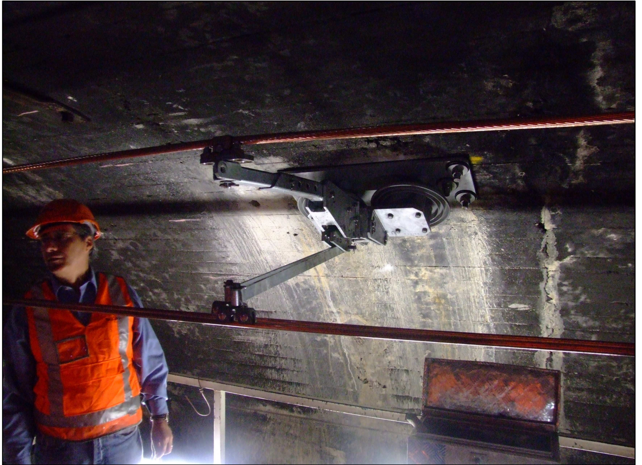
Figure 5 - Lateral View of Mk-3 Tunnel Cantilever
